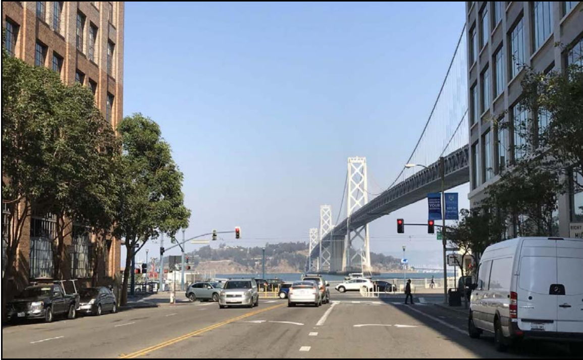
Figure 14a. Existing View of Project Site Looking East from Harrison Street
